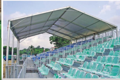
High Stand Column with Side Tension Bracing
