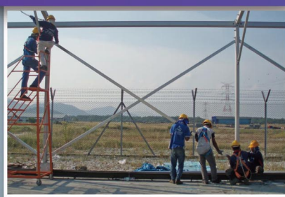
Cross Tension Bracing
