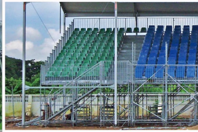
High Stand Column with Side Tension Bracing
